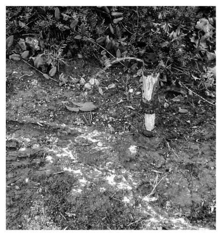
The sprinkler head pictured continues to dribble water long after the valve has been shut off. The ruts in the soil as a result are obvious. The remedies are to install a sprinkler head with a check valve, raise the head, or shore up the slope around the head with large drain rock.
