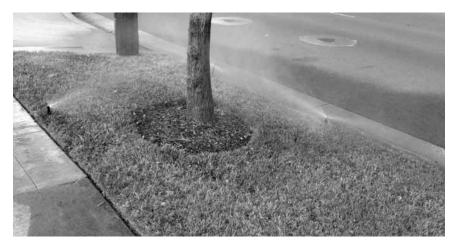
The street and driveway are noticeably wet. The mist produced from these sprinkler heads has been caught by the wind. The water pressure needs to be reduced and/or the heads replaced.
