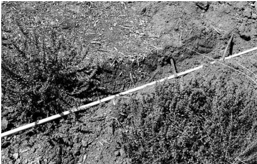
Inline emitter tubing being installed a couple inches below ground. Courtesy of Camrosa Water District.
