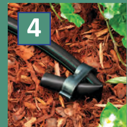
Dripline end figure 8 can double as a flush-out valve
