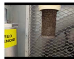
Plugged screen filter prior to blowdown valve
