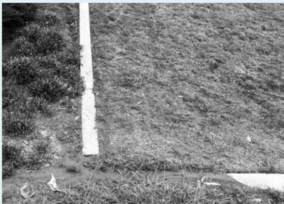
This slope needs pulse irrigation. Rills at the top of the photo and a buried mower strip at the bottom mean that the slope is getting water faster than it can accept it.
