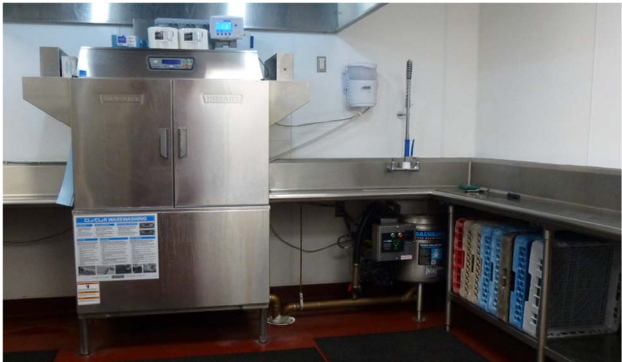
Figure 18. Casper—Dishmachine with Pre-rinse station and scrap collector
