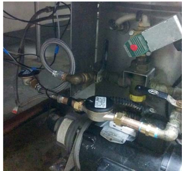
Figure 21. Conference Center—Utility hose/sprayer water meter (left); collector water metering (right)
