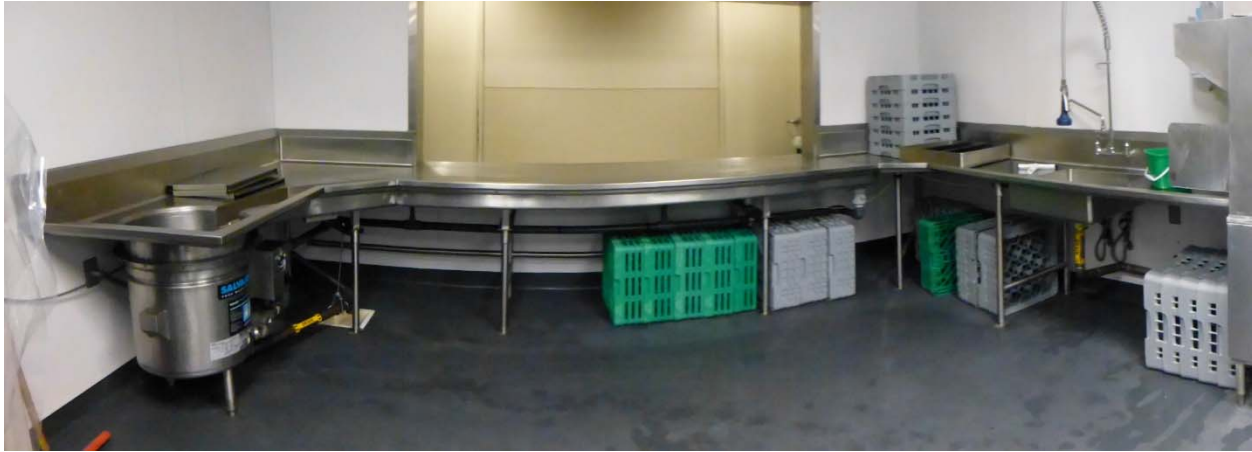
Figure 24. Arrillaga—Renovated drop-off window, trough-fed collector and pre-rinse station
