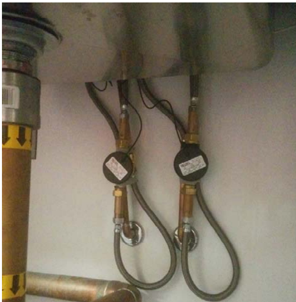
Figure 25. Arrillaga—Water meters on pre-rinse spray valve (left) and on scrap collector (right)
