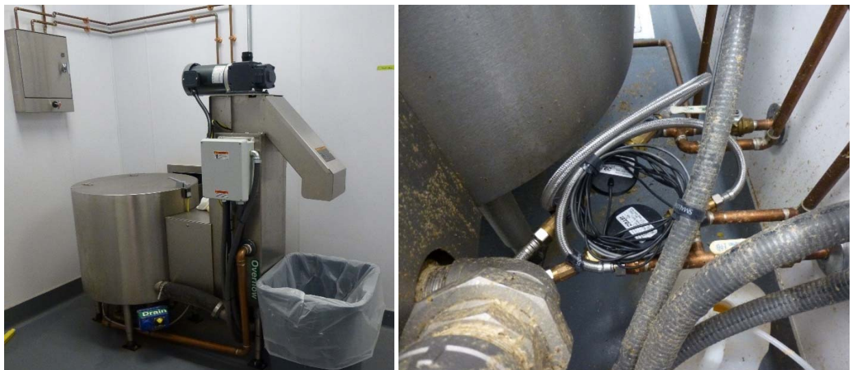
Figure 29. Corporate Café 4—Pulper system (left); hot and cold water meters connected to pulper (right)
