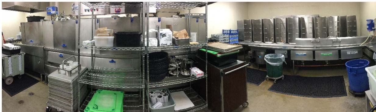
Figure 20. Conference Center—Flight Dishmachine (left) and pre-rinse area (middle in the background)
