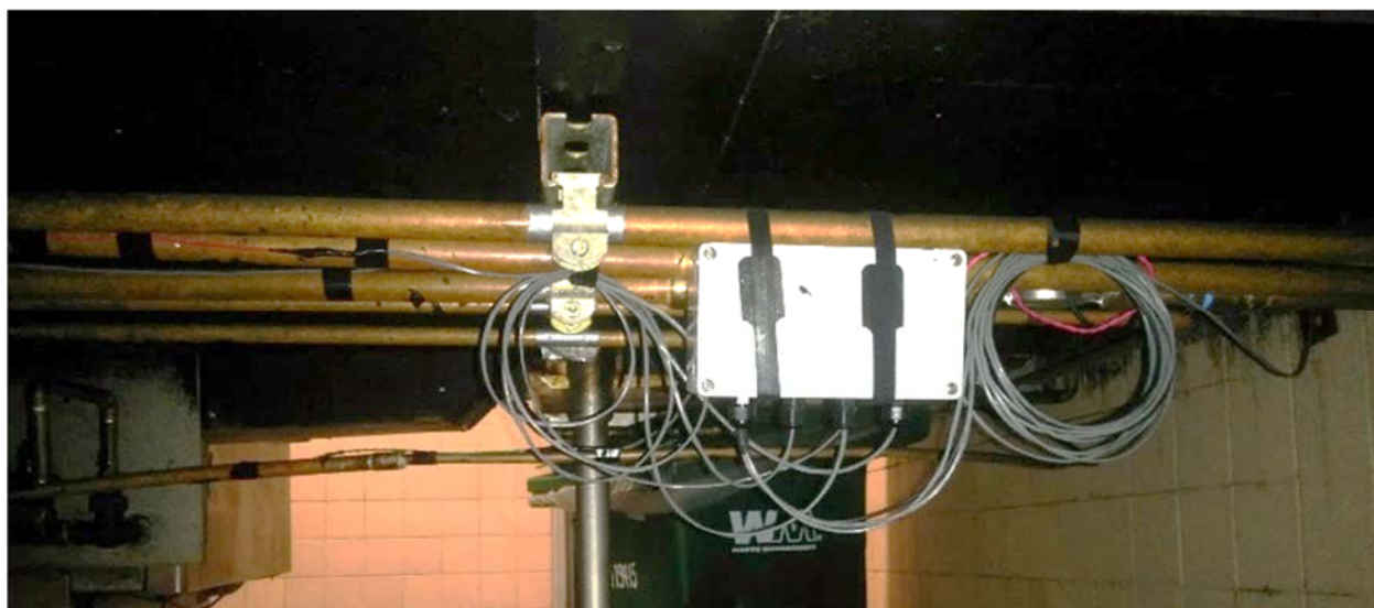
Figure 15. Marriott—Datalogger enclosure and in-line water meter
