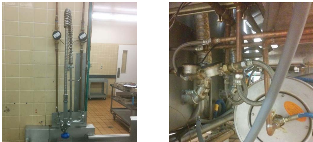
Figure 13. Belas Hall—PRSV and water meters installed (left); water meters installed on hose reel (right)
