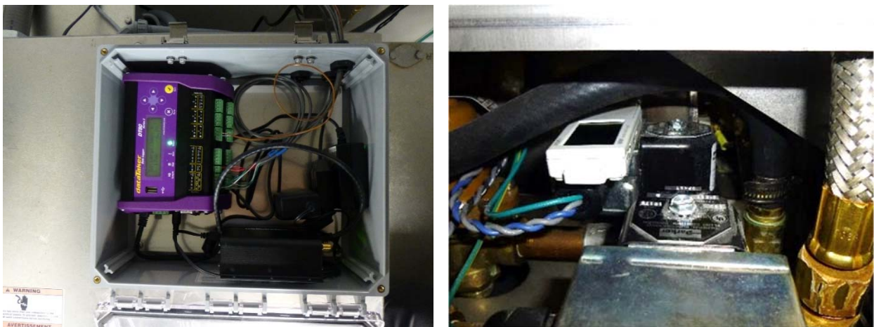
Figure 31. Corporate Café 4—Datalogger in enclosure (left); logger on dishmachine rinse solenoid (right)
