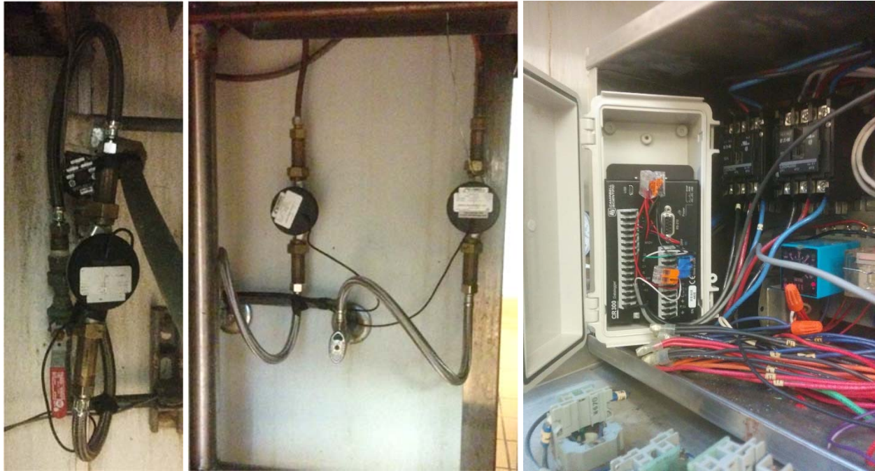
Figure 11. Schwab—Disposer water meter (left); PRSV water meters (center); data logger (right)
