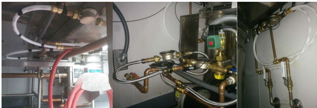
Figure 27. Corporate Café 3—Metering for hose (left), scrap collector (center) and pre-rinse sink (right)
