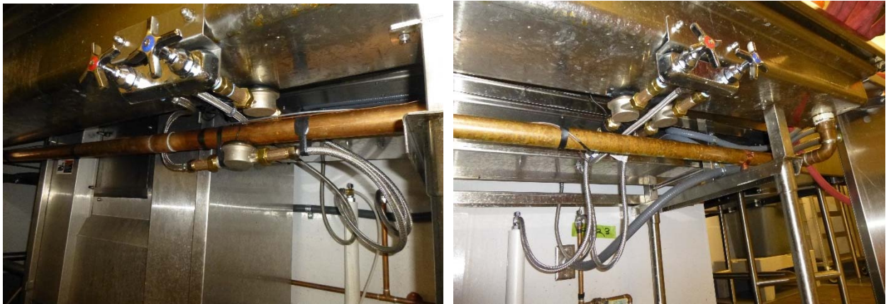
Figure 30. Corporate Café 4—Left PRSV_1 water meters (left), and right PRSV_2 water meters (right)
