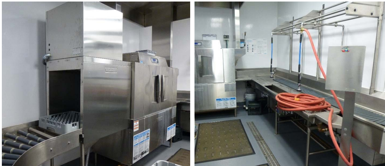
Figure 28. Corporate Café 4—Dishmachine (left); pre-rinse station with 2 PRSVs, trough and hose (right)
