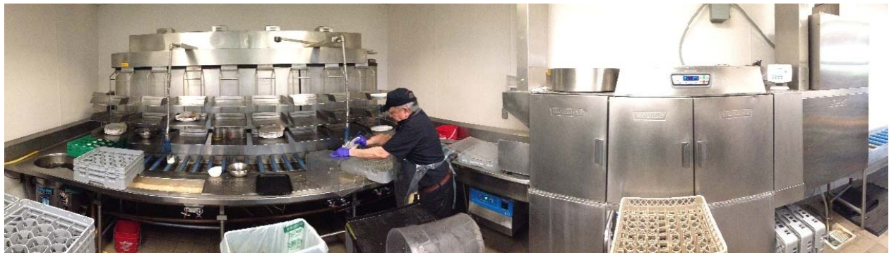
Figure 22. Arrillaga #4—Original pre-rinse area with tray accumulator prior to renovation
