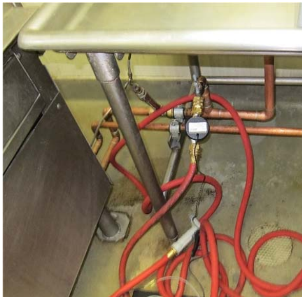
Figure 21. Conference Center—Utility hose/sprayer water meter (left); collector water metering (right)
