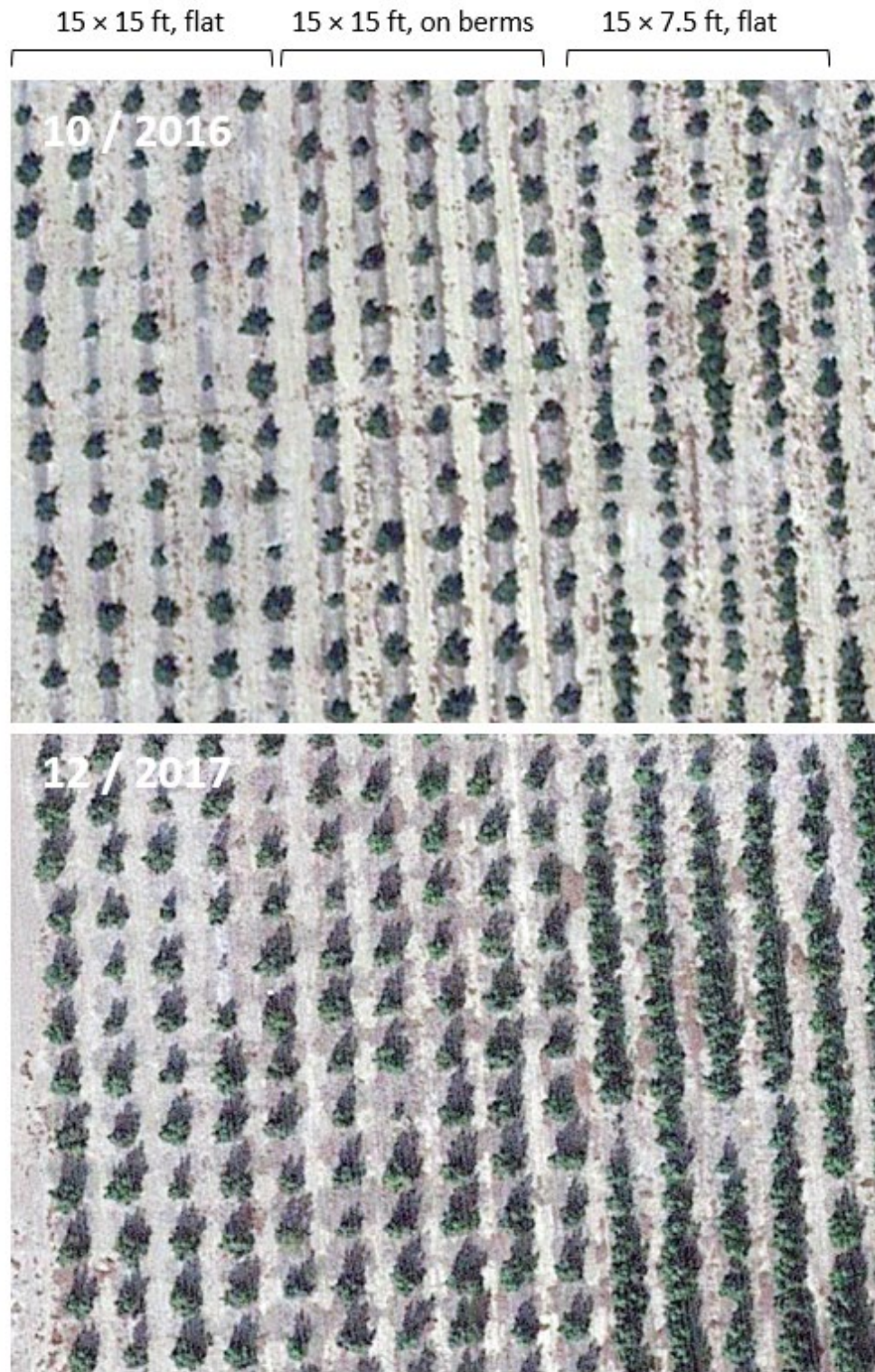
Fig. 2. Aerial photographs of the study site at Pine Tree Ranch, Santa Paula, California, in October 2016 and December 2017, obtained from Google Earth Pro. The soil berms are clearly visible in the upper image from 2016.
