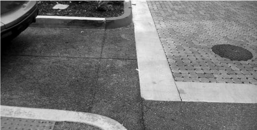
Both the porous concrete and pavers will need periodic vacuuming or sweeping to maintain efficiency.
