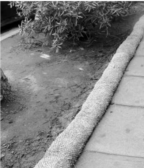
Fiber rolls are protecting the sidewalk from the DG mulch. The DG should be removed. Not only does it have a tendency to travel on slopes, but it is easy to compact and quickly produces runoff. DG is ill advised on slopes.
