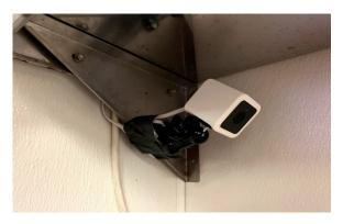
Figure 2: Camera mounted onto the corner strut.
